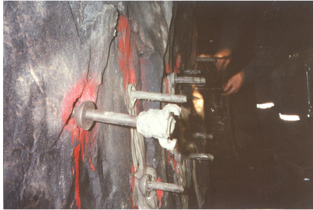
Grouted pipe bolts (0.4 w/c grout)
