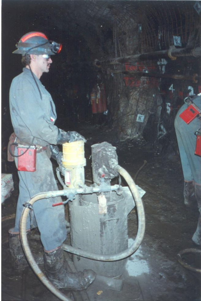
Mixing cement grout in a Speidel pump/mixer
