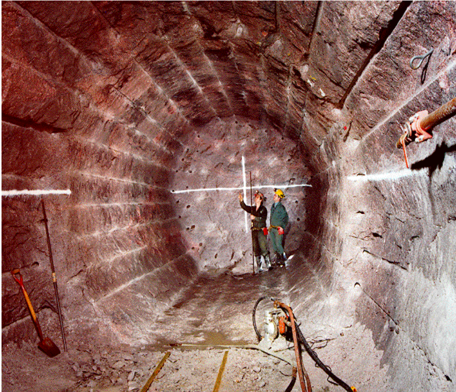
In good conditions
