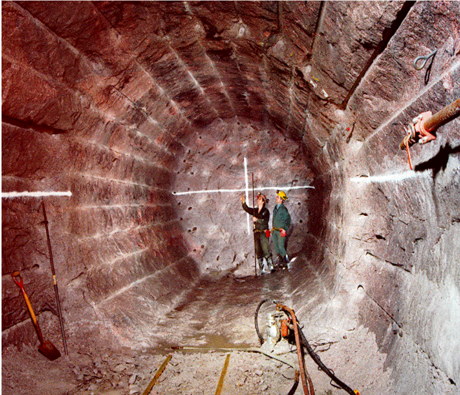
In good conditions
